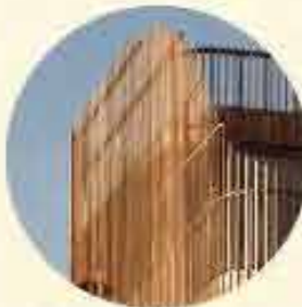
Self-shading prefabricated timber facade
